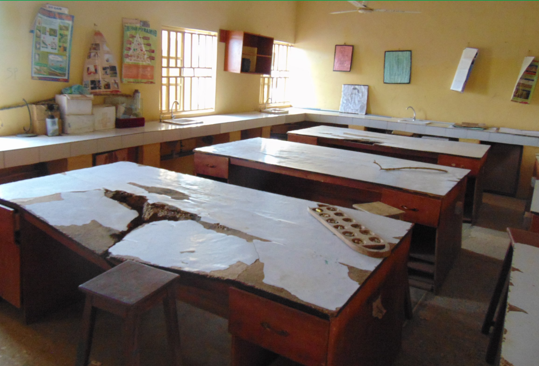
Broken table at the technical workshop at JSS Karshi, FCT, Abuja
