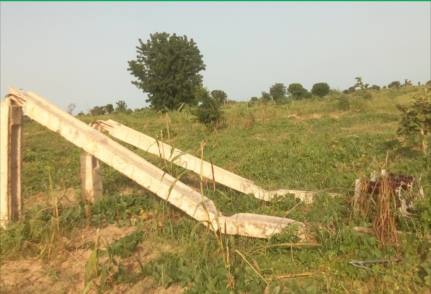
Two of the fallen electric poles in Ungwabawa, near Birnin Kebbi, Kebbi State. The electrification project had been abandoned for nine years.
